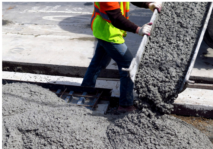
A worker pouring concrete during construction of a sidewalk in Washington, DC.
