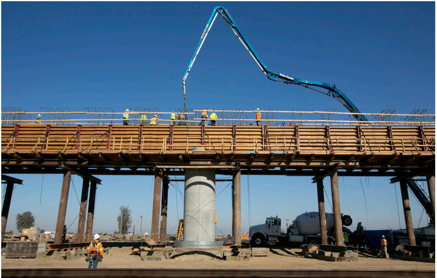
Workers pouring concrete onto an elevated section of a high-speed rail line near Fresno, California.
